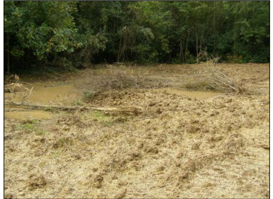
Woody debris and plants added to wetlands during construction.
