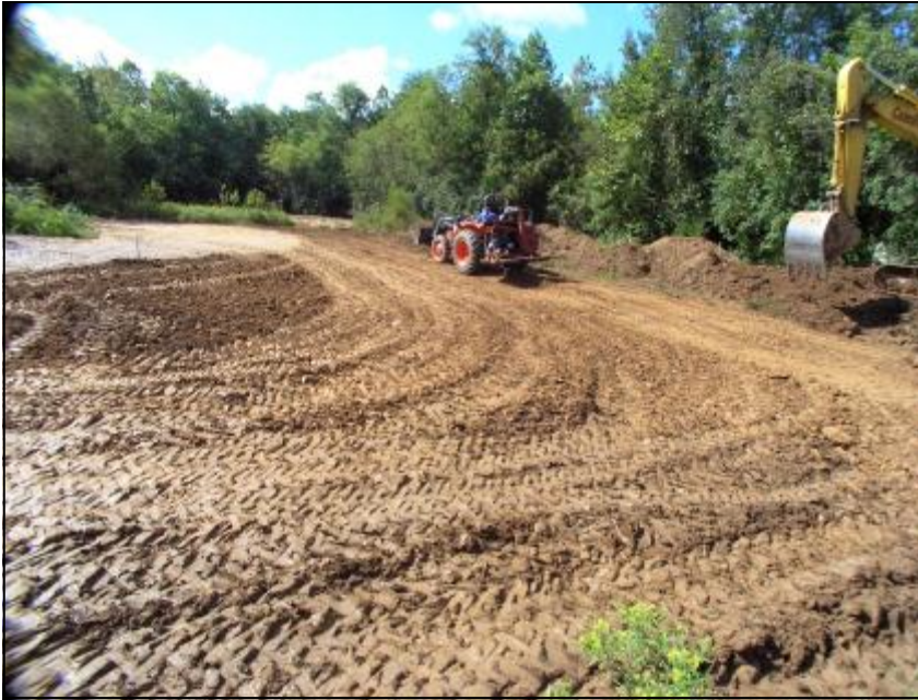
Above: Compaction of clay soils in wetland. Below: Smoothing and shaping of wetland.
