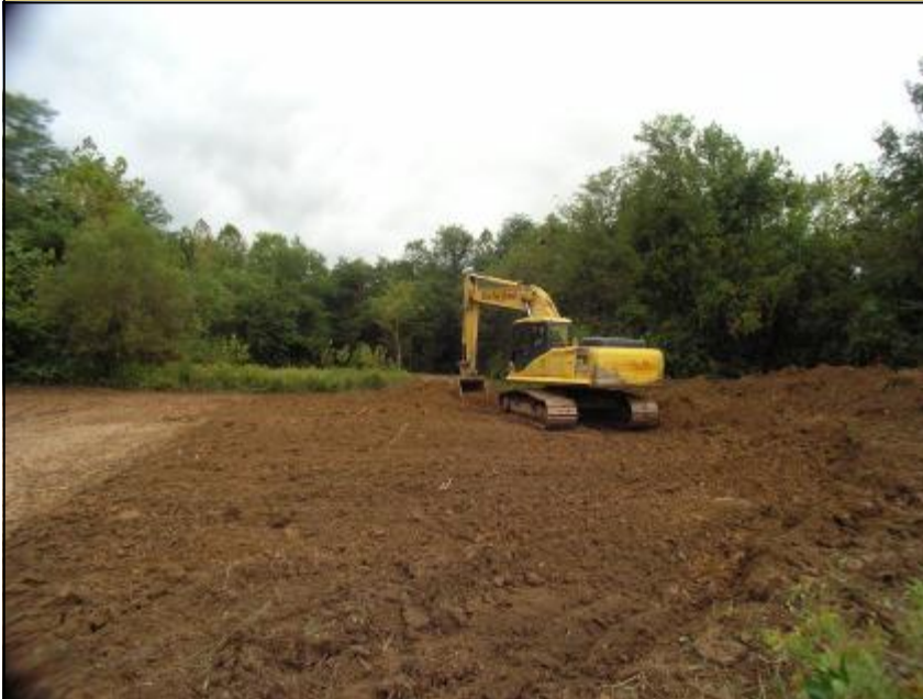
Above: Compaction of clay soils in wetland. Below: Smoothing and shaping of wetland.
